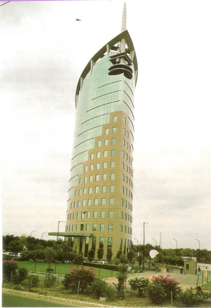
DLF Gateway Tower, National Highway 8, Gurgaon
