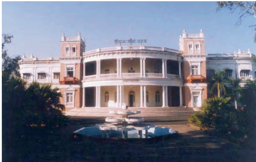
Figure 1. Front View of the Minto Hall (Courtesy: Authors)
